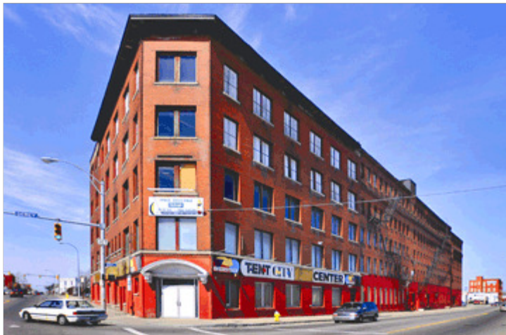
Winn Development hopes to redevelop the former Tent City sporting goods store at the corner of Dewey and Lyell avenues in Northwest Rochester in to 83 apartment units, an estimated $23 million project.
